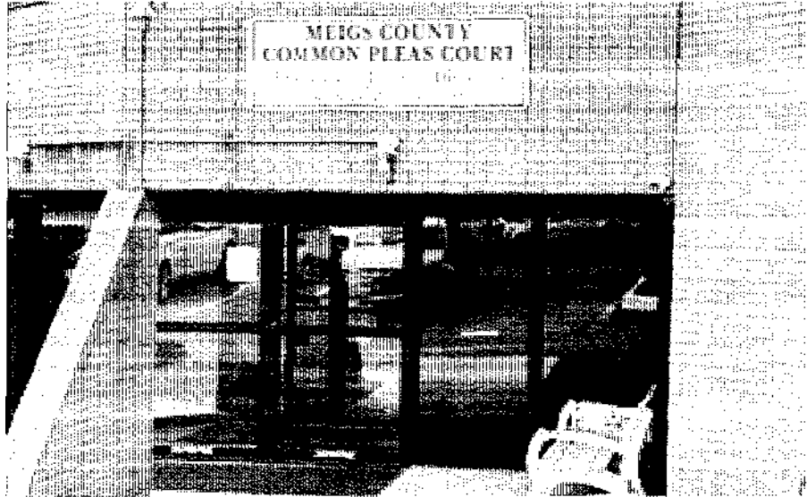
(112 East Memorial Drive, Ground Floor, Pomeroy, Ohio - Physical Building Address)
